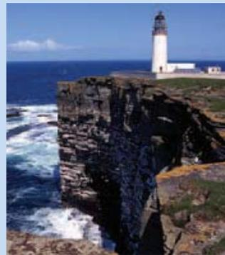
Noup Head Lighthouse (built 1898) was the first in Scotland to use mercury floatation in the revolving carriage. The tower is 24m high and the light now flashes every 30 seconds. The light was automated in 1964 when a new lens was installed and, in 2001, solar power replaced gas, with the use of 36 solar panels.
